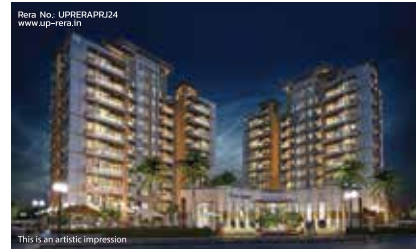
REERA No. UPRERAPRJ224 www.up-dera.in This is an artistic impression ELDECO LUXA SITAPUR ROAD, LUCKNOW
