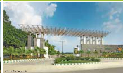
Actual Photograph ELDECO SHAURYA BINOR ROAD, LUCKNOW
